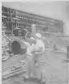
H. A. Mathiason points out a detail of Hospital construction to G. Hiemstra.
